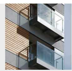
This residential installation features an Opal balustrade with stainless steel handrail on the balconies, an Opal balustrade on the stairs and perforated panels to the Juliet balconies. The chosen design combines elements of the Opal and Onyx ranges.
